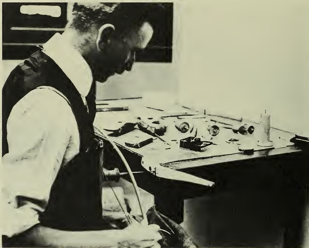
FIG. 76.—Wampum making: Perforating a roughly shaped bead.
